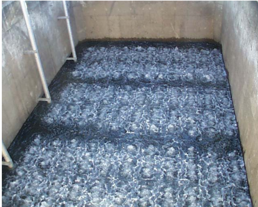
FIGURE 1 - TYPICAL AERATION GRID PATTERN
